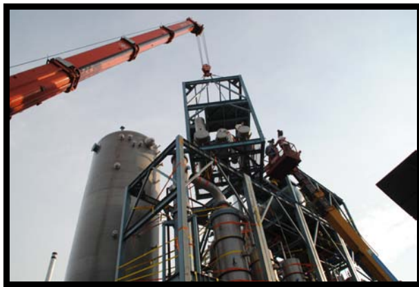
View of pre manufactured skids being stacked
