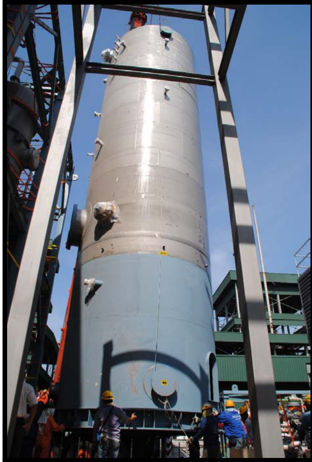
View of distillation column being installed
