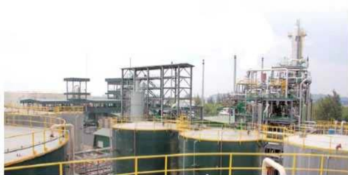
Mission's Biodiesel Refinery
